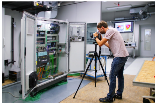
WKC - Test laboratory - Heat measurement
